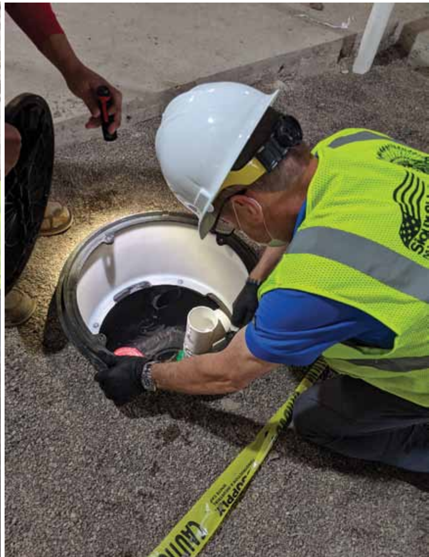
Armstrong checking an installation of one of their grease interceptors at the Footprint Center in Phoenix where the Suns basketball team plays.
