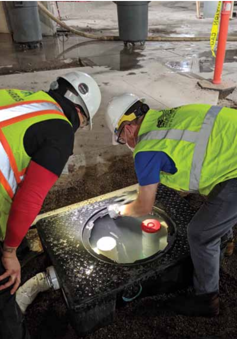
Armstrong checking an installation of one of their grease interceptors at the Footprint Center in Phoenix where the Suns basketball team plays.
